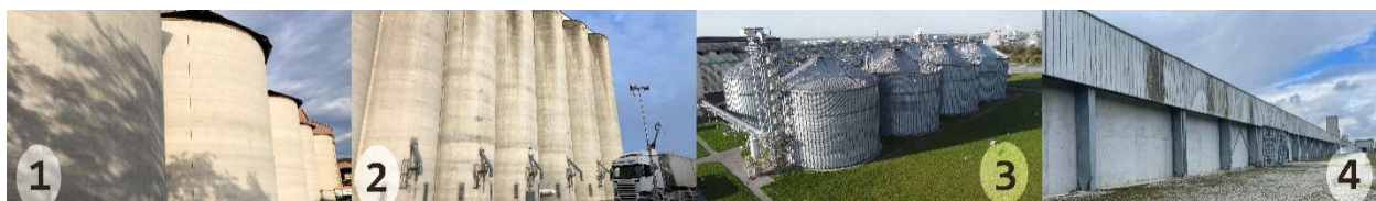
Fig. 3. Four treated storage systems located in France: 1–Baziège, concrete bins, durum wheat, no active diffusion or recirculation; 2–Roncenay, conical bottom concrete silos, peas, active gas diffusion with recirculation; 3–Pomacle, metal bins, wheat, active diffusion, no recirculation; and 4–Buchères, ground sheds, wheat, injected gas, no recirculation, and no tarping.
